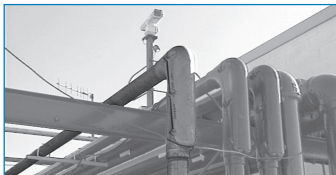
TYPICAL CLASS I, DIVISION 2 RIGID CONDUIT INSTALLATION.
