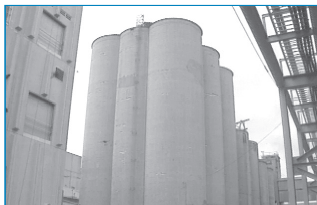
GRAIN ELEVATOR — CLASS II, DIVISIONS 1 AND 2.
